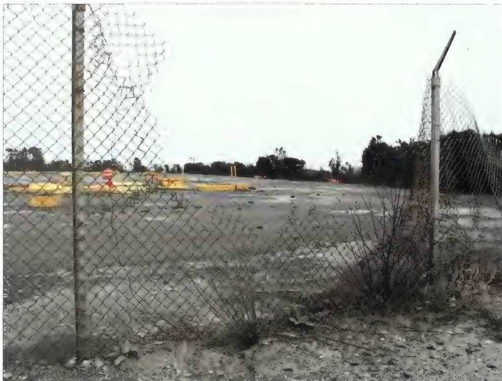
Figure 4.28. View looking southeast across Missile Magazines, NIKE launch site. The Army installed an inner security fence around the Missile Magazines as a component of the launch site's security upgrades to use Hercules missiles fitted with nuclear warheads. The inner fence is presently extant with chain-link sections attached to H-shaped posts and is in fair to poor condition (Olmsted Center, April 2008).
